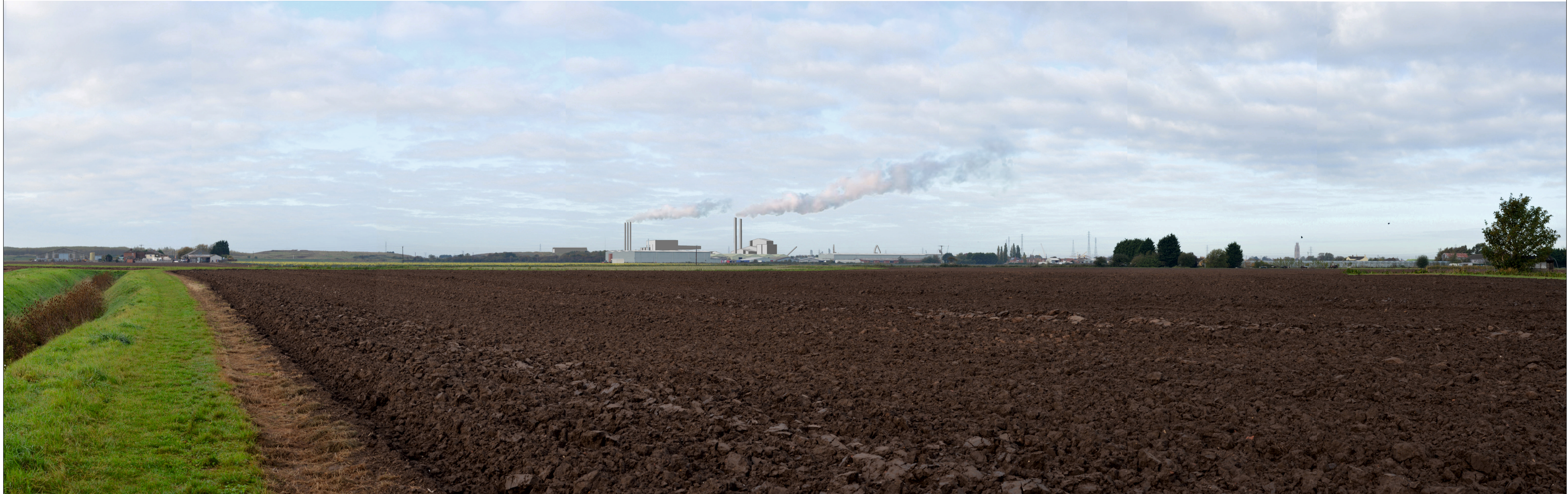
View 3: Photomontage view of the proposed Facility at Year 1 illustrating stack plumes at 'maximum' length (see notes below)
